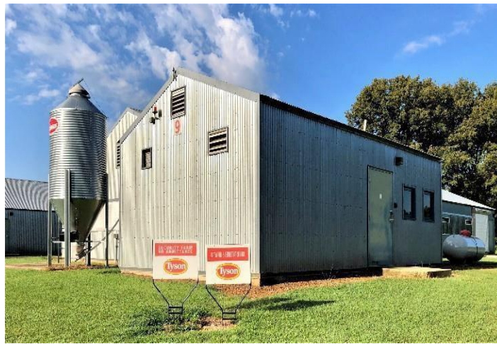
Figure 16 – The Tyson Facility at UTM
