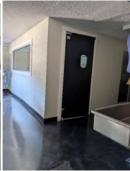
Figure 10 f - inside of classroom upgrades
