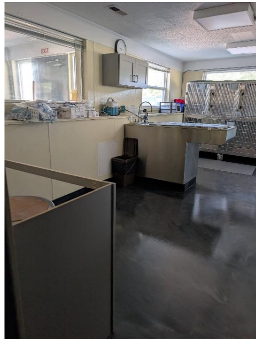
Figure 10 h - inside of classroom upgrades
